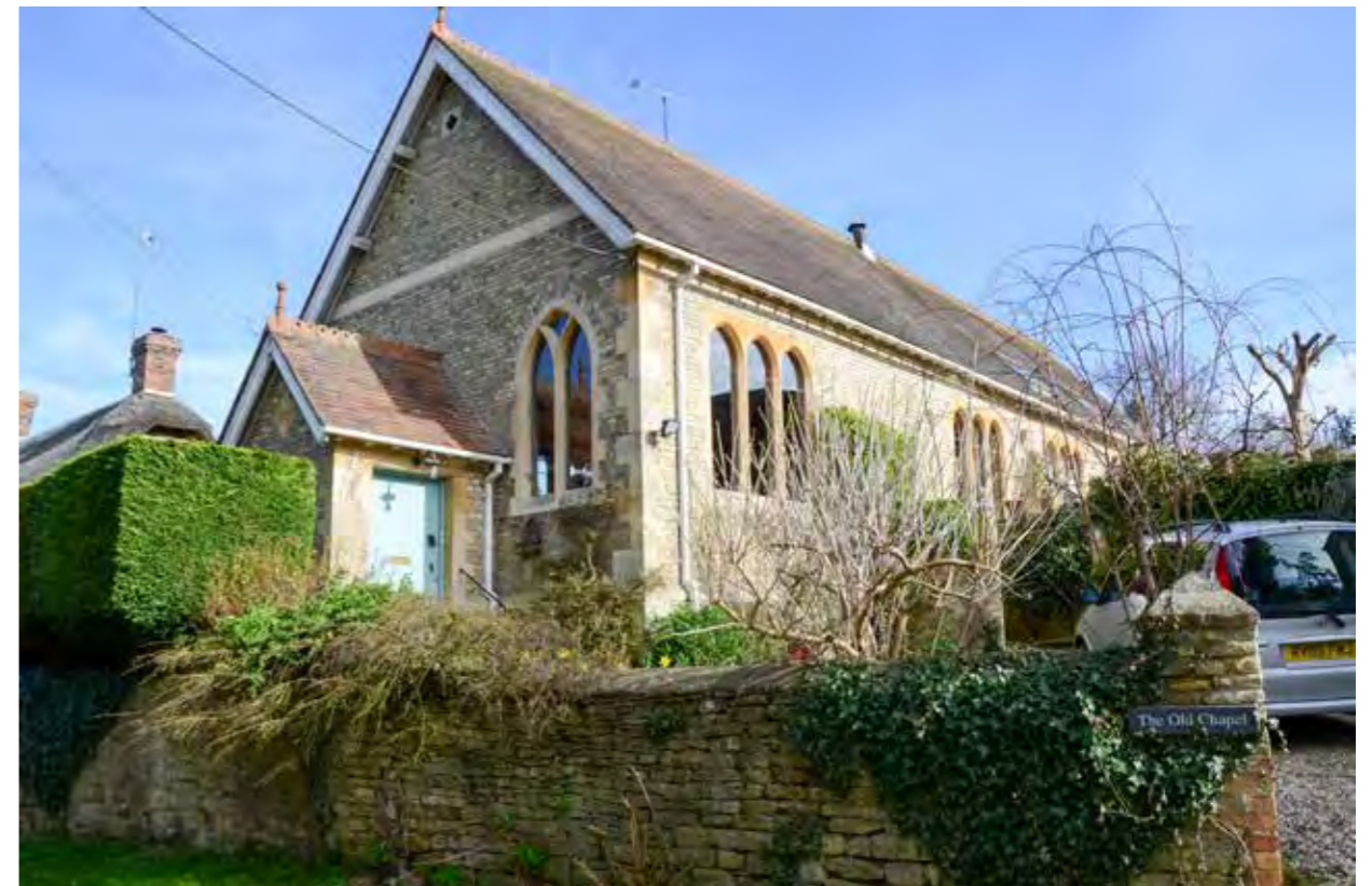
B. Old Chapel, Mill Lane
