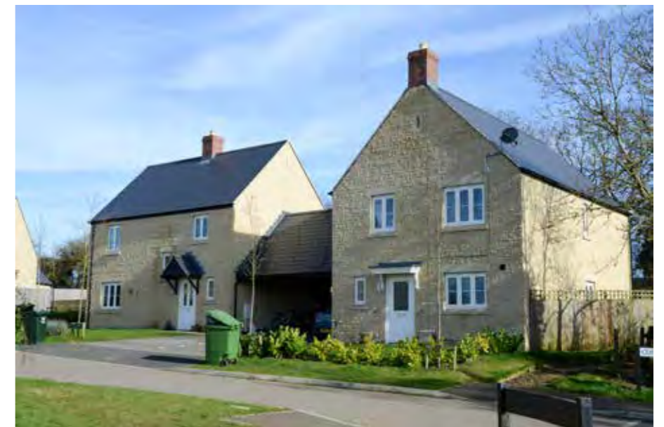
Recent housing at the western rural exception site on the edge of the village
