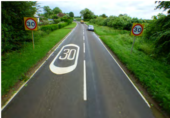
Centre lines and unchanged carriageway widths encourage speeds
