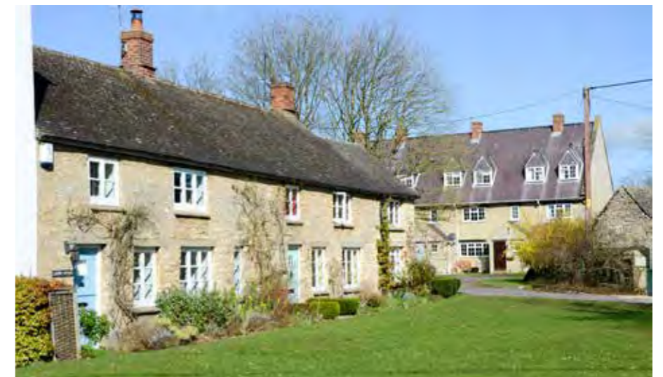
More recent development (rear) has favoured dormer third storeys which are out of scale with the historic development within the village (fore)
