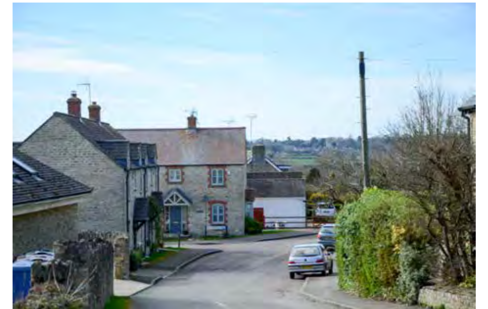
Recent housing along Orchard Lane is a good example of the local vernacular
