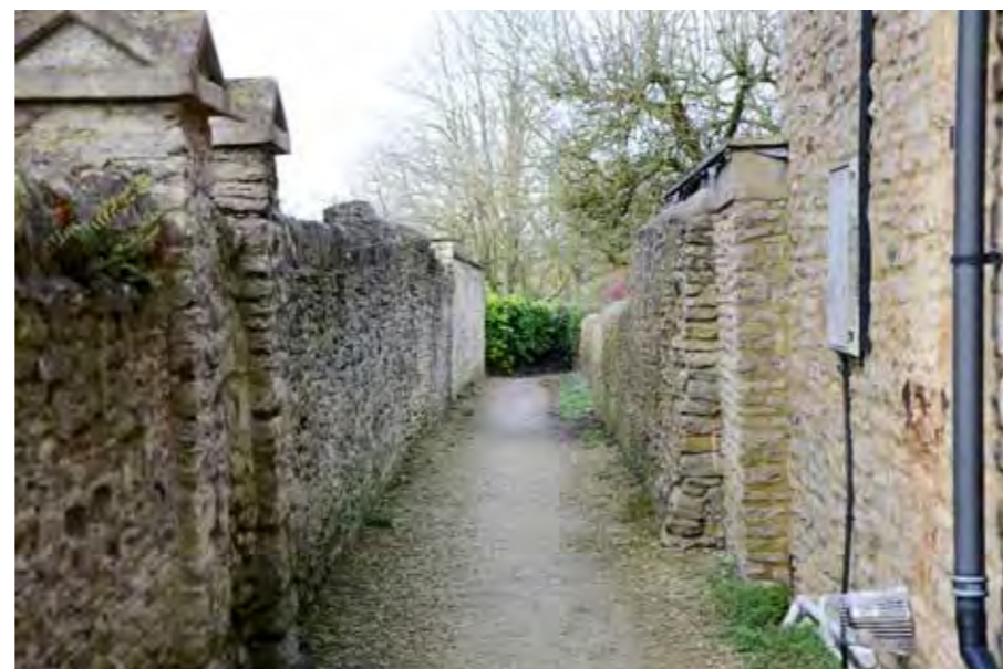
Historic lanes lined by limestone rubble walls
