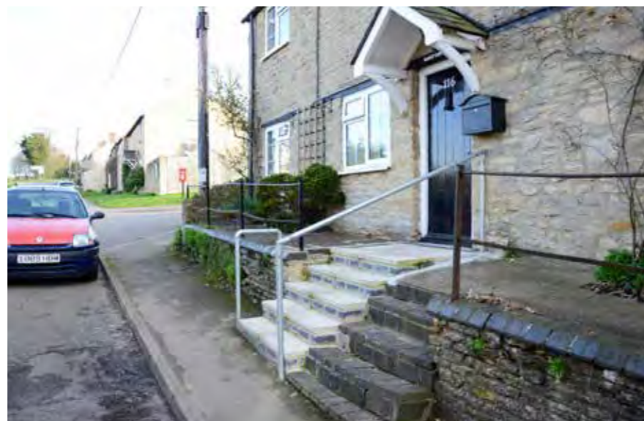
Poor detailing and unsympathetic design can detract from the character of the public realm
