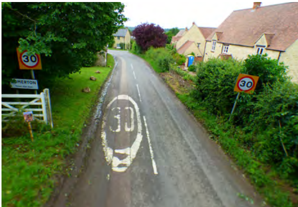
Entry to Somerton marred by road markings
