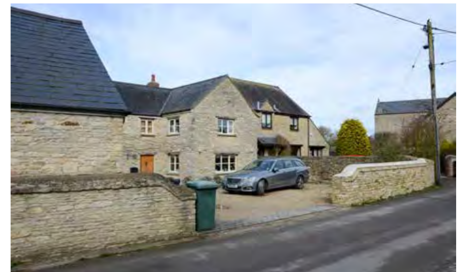
Recent interventions to the stone wall and the driveway are sympathetic to the building and character of the village
