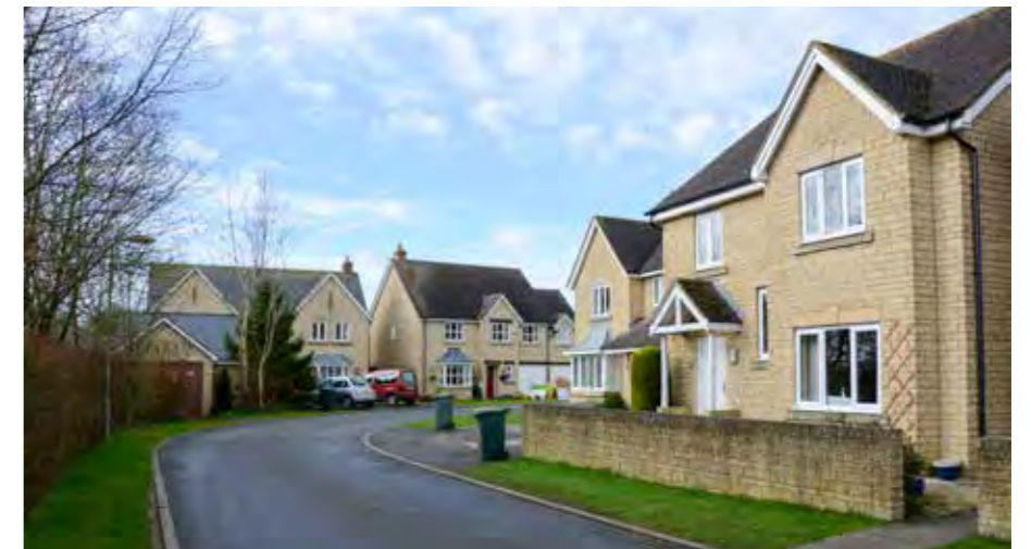
More recent development lacks the detail and finish of the local vernacular
